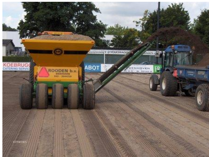
Secondary drainage installation
