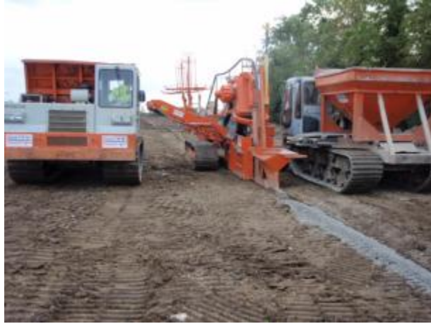
Drainage installation
